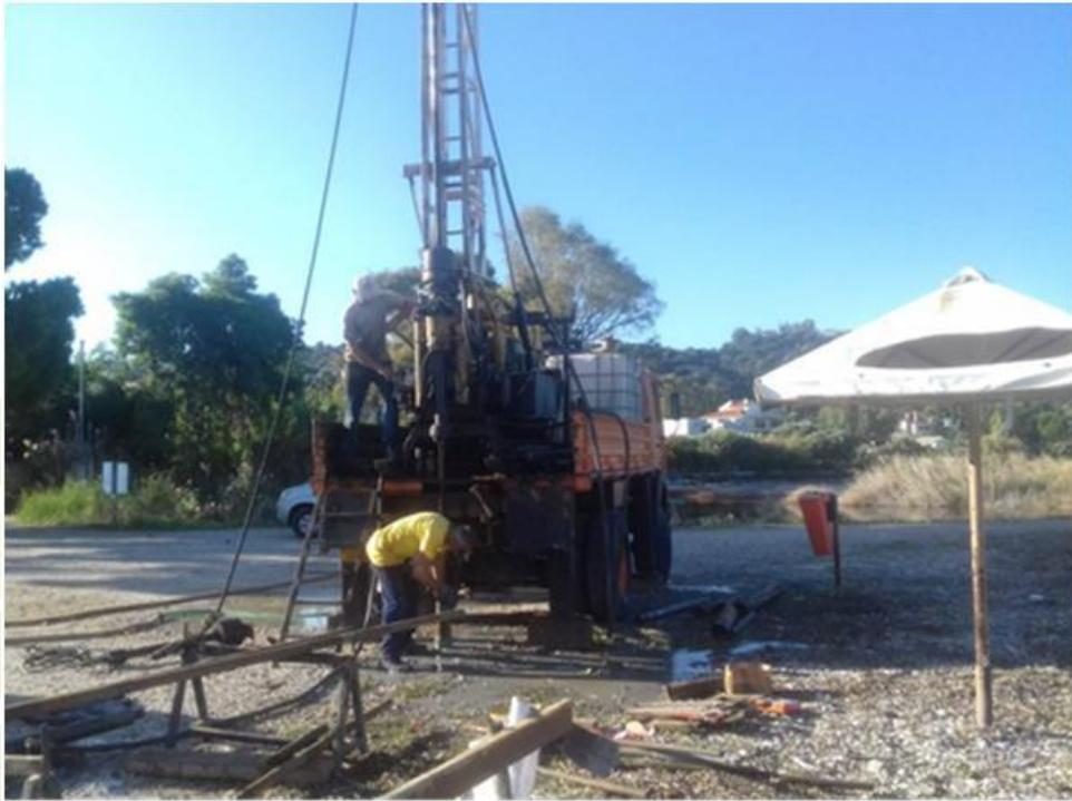
**Figure 3.24:** BOYLES rotary drilling used for the drilling of boreholes
